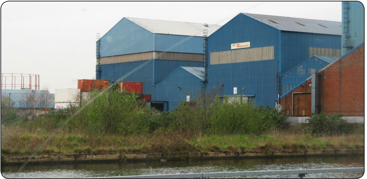
Former Industrial Building at Meridian Water being re-purposed as Meridian Works to provide a meanwhile use
