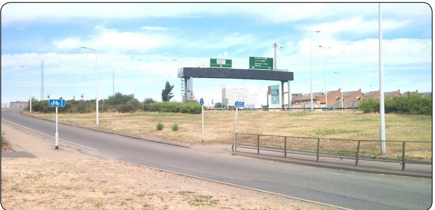
North Circular Road and Slip Road
